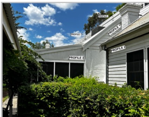
Plate 22 – 13 Gwydir Street; various cladding profiles on rear eastern side Source: Author
