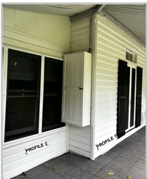
Plate 24 – 13 Gwydir Street; various cladding profiles on front wall; Source: Author
