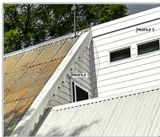
Plate 25 – 13 Gwydir Street; various cladding profiles on upper floor area, rear eastern side; Source: Author
